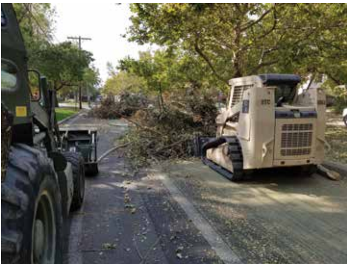
The 1457th Engineer Battalion conducts debris removal in Northern Utah neighborhoods during windstorm debris cleanup in August 2021.
