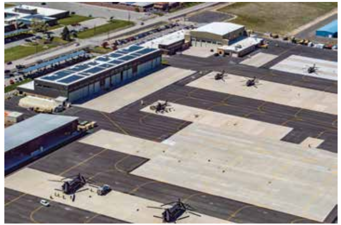
Aerial view of the Utah National Guard Army Aviation Support Facility located at the South Valley Regional Airport in West Jordan, Utah.
