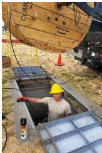
Members of the 130th EIS stand in front of the FedEx field "Solar Man" after redeploying the JICC mobile communications asset in the press box of the stadium during the 59th Presidential Inauguration. Tech. Sgt. Lamont Class guides a 48-strand fiber optic cable through the underground conduit system at Portland Air National Guard Base, Oregon, August 2020. Senior Airman Ben Meads, Tech. Sgt. James Gibson, Tech. Sgt. Travis Jemmett, and Master Sgt. Brandon Musgrove deploy a low VHF tactical antenna mast for JICC direct Line of Sight radio communications for Washington D.C. Capital Quick Response Force. Staff Sgt. John Geister completes pole-rescue training at Roland R. Wright Air National Guard Base, Salt Lake City, Utah, October 2020.
