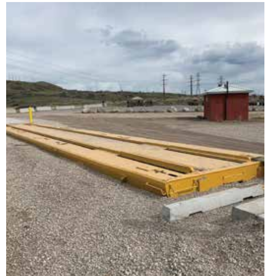
The Construction Facilities Management Office completed the rail-load training facility at Camp Williams, Utah, in May of 2021. The facility will increase the Utah Army National Guard's capability to train unit movement officers and rail-load teams.
